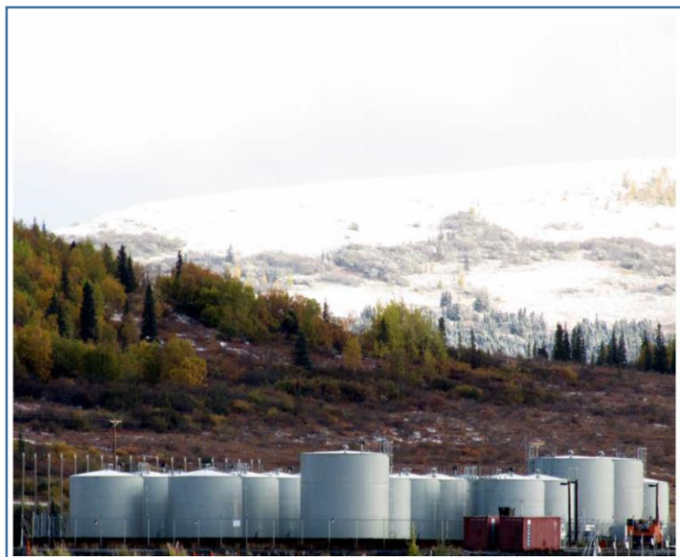
Figure 10 Unalakleet tank farm. Photo courtesy of Unalakleet Economic Development Plan 2014-2019.
